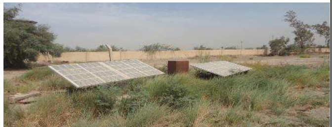
4- Using Solar renewable energy
