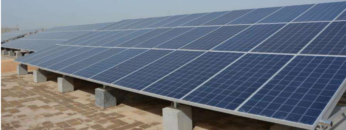
5- Using Solar renewable energy
